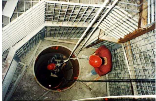
Figure 4. Receiving shaft: Putting geophones in the pyroclastic formation basement rock.
